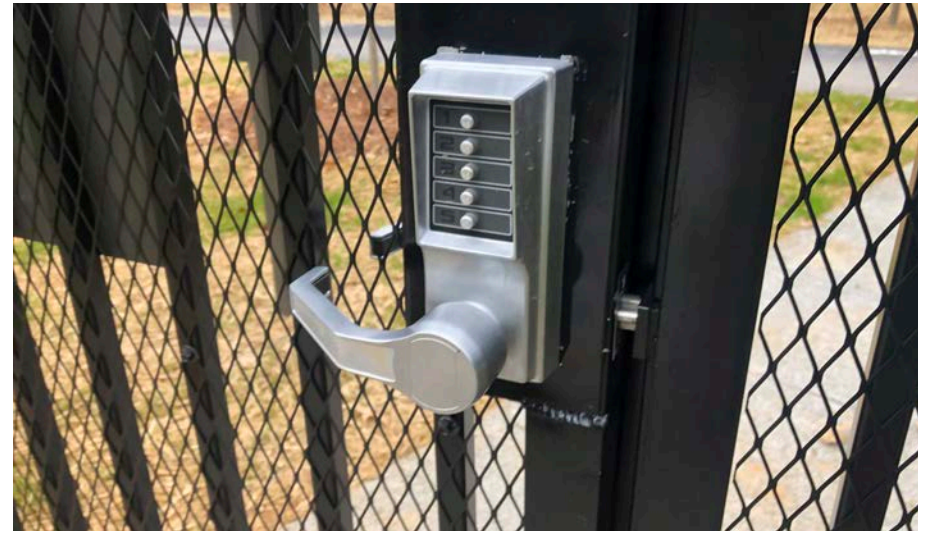
Example of coded access gate for multi-family housing along the PCG in Brookhaven, GA
