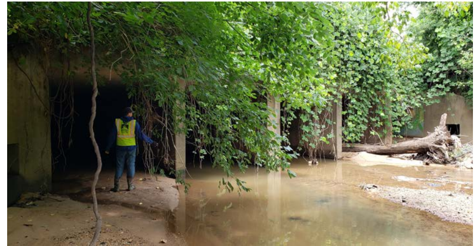
Existing five box-culvert under Chamblee Tucker Road, facing northwest. A flood study is advised to confirm that the eastern most box may be reconfigured for a 10'-0" wide multi-use trail.
