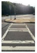
The photo to the left shows an ADA ramp that should be approved. There is a 3-4" displacement at its base that we cannot cut. Because we do not provide concrete construction services, this is not work we can complete. It requires the attention of a general contractor or your public works department.
