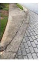
This next photo shows a ramp cut that is included in this repair offer. We will cut the concrete where it connects to curb to create a flush joint between the two surfaces.
