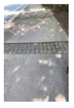
The photo to the left shows a repair that we can make as part of this repair offer. We will cut the concrete where it is higher than the brick pavers to create a flush joint between the two surfaces.
