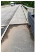
The photo to the left shows sidewalk that should be replaced against a bridge. We avoid cutting into bridge structures since they are frequently part of the structural support. Because we do not provide concrete construction services, this is not work we can complete. It requires the attention of a general contractor or your public works department.
