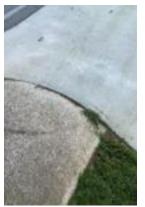
The photo to the left shows a chipped joint that can/should be filled. We do not provide this type of work because it can normally be done less expensively by our own customers public works staff with materials purchased at local hardware stores.
