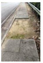
This next photo shows sidewalk that is missing. New concrete should be added to complete the walkway. Because we do not provide concrete construction services, this is not work we can complete. It requires the attention of a general contractor or your public works department.
