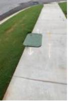
The photo to the left shows an example of an uneven utility. All utilities within the profile of a sidewalk should be flush with the walking surface. This is an issue that we can not resolve. It is something that should be corrected by your utility vendor or public works department.
