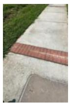
The photo to the left shows brick pavers in the sidewalk that are too high and need to be reset flush. This is not work that we provide. It will require the attention of a general contractor or your public works department.
