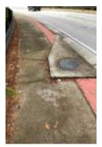
The photo to the left shows sidewalk that should be replaced around a catch basin. We can sometimes cut the basin cover if the position of the manhole allows us to cut an ADA compliant slope, and the displacement is 1" or smaller. Neither apply in this case. Because we do not provide concrete construction services, this is not work we can complete. It requires the attention of a general contractor or your public works department.
