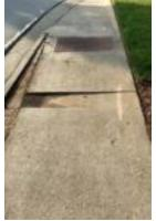
This next photo shows another area where sidewalk should be replaced with new concrete instead of repaired. It is bad policy to cut and fill strips of concrete in a sidewalk. They always sink and crack and do not last very long. Because we do not provide concrete construction services, this is not work we can complete. It requires the attention of a general contractor or your public works department.
