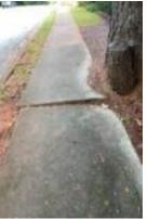
The photo to the left shows a displacement that is too big for our repair process. It is well over 2" high. If we cut away the high concrete it will leave a slab that is too thin and susceptible to breaking. This sidewalk should be replaced with new concrete. Because we do not provide concrete construction services, this is not work we can complete. It requires the attention of a general contractor or your public works department.
