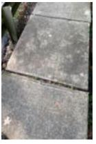
The photo to the left shows a wide gap between sidewalk panels that can/should be filled. We do not provide this type of work because it can normally be done less expensively by our own customers public works staff with materials purchased at local hardware stores.
