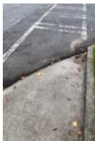
This next photo shows asphalt that is too high where it connects to the concrete of an ADA ramp. We can but do not normally cut asphalt because we do not work the cost of traffic control into our pricing or possess the ability to control traffic. This will require the attention of your own public works department.
