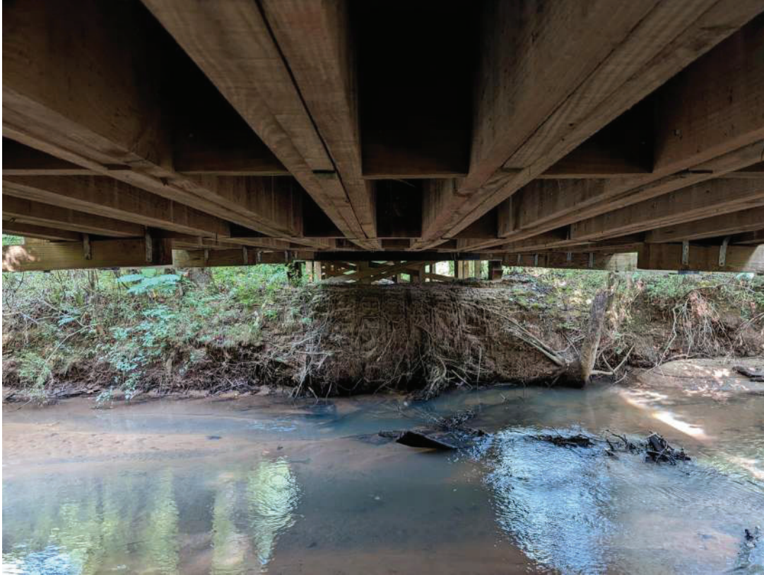
Photo 2 – Bridge #1 Overall Photo (Below)
