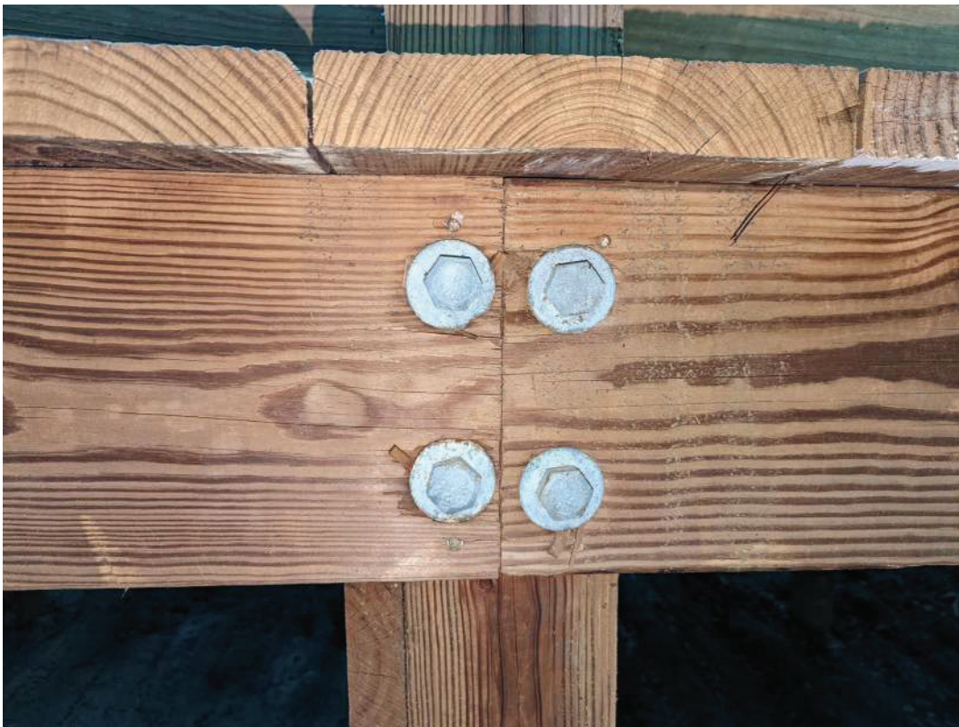
Photo 8 – Boardwalk Post to Beam Connection (Typical)
