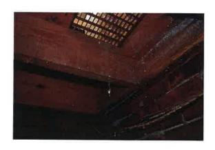
2x8 Floor joists are over spanned 36" average. Sagging entry level floors have been supported via multiple screw jacks in the Crawl/basement. However, 2<sup>nd</sup> floor joists would require removal of all ceilings, electrical and plumbing to facilitate 'sistering' of all joists.
