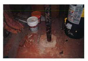
Retrofit steel bracing is supporting over-spanned floor joists, inadequate beams, and a suspended concrete slab. This level is rendered effectively unusable although the bracing employed is still insufficient.
